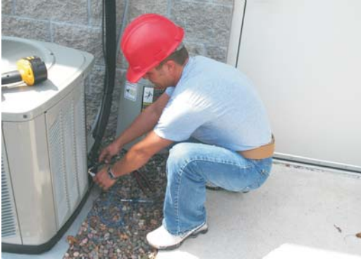
Installation of the voltage monitoring relay and tamper switch is quick and easy.
