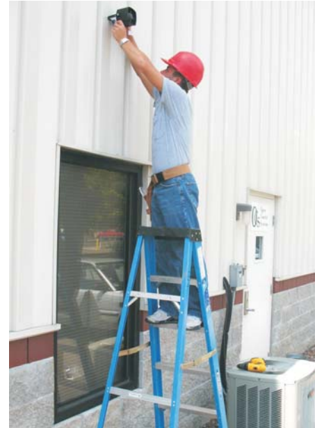
Extremely loud 118 dB siren can be mounted outside or inside the building.
