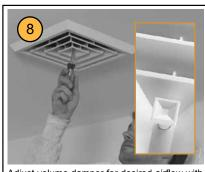
Adjust volume damper for desired airflow with a straight-blade screwdriver or insert included handle through the access hole in the center of the grille and snap firmly in place. Handle may be removed or left in place.
