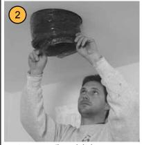
Pull flexible duct through hole.
