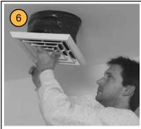
Push the diffuser and flexible duct into opening until grille contacts the ceiling. Rotate unit until it is parallel with walls in the room.
