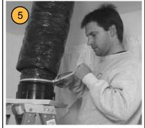
Slide duct over a collar and secure using tie wrap (provided). Tighten using tie wrap tool or pliers
