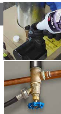
▲ Force pump drain line injection
